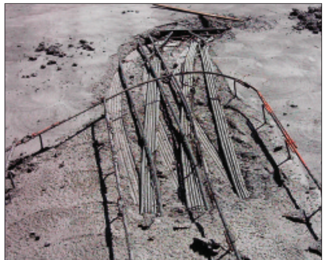
Left: Slab penetrations too close to anchors can result in blowouts. Right: This horizontal blowout resulted from tendons that were curved in a very tight radius. On the left side of the photo, the imprint of the tendons prior to stressing can be seen approximately 12 inches away from their current location. During stressing, the tendons straightened and the concrete in the curve was unable to resist the localized lateral thrust.
