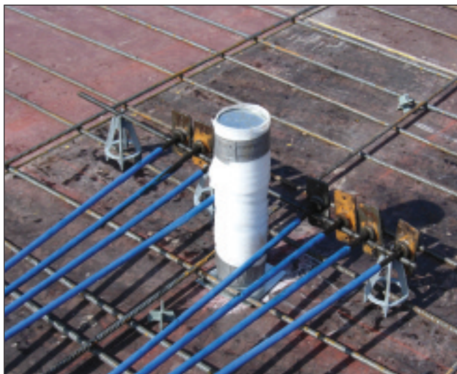
Left: Slab penetrations too close to anchors can result in blowouts. Right: This horizontal blowout resulted from tendons that were curved in a very tight radius. On the left side of the photo, the imprint of the tendons prior to stressing can be seen approximately 12 inches away from their current location. During stressing, the tendons straightened and the concrete in the curve was unable to resist the localized lateral thrust.
